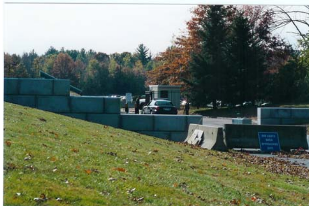
Plas-Crete blocks made by Conigliaro Industries are used as force protection at the Massachusetts National Guard Headquarters in Milford, Mass.
